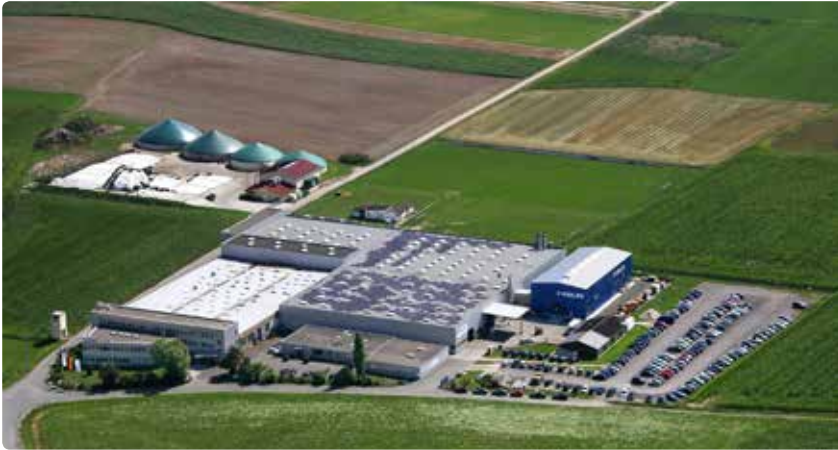
Resource-efficient: photovoltaic electricity and heating with biogas waste heat
