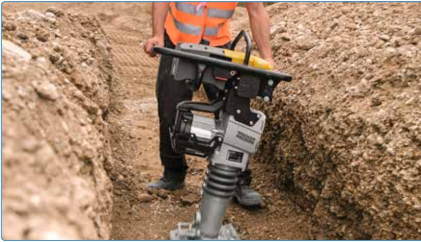
Working emission-free with the battery rammer AS50e.
